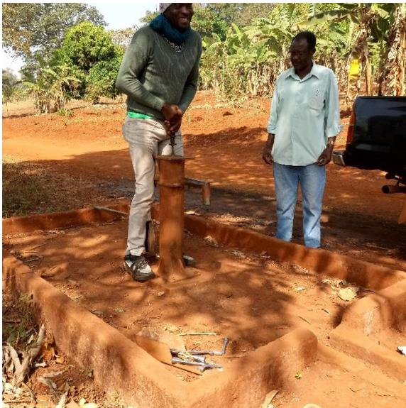
Testing if the cylinder is connected
