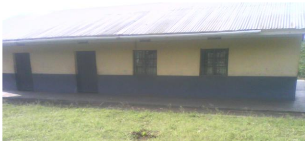
Health expansion: Above; Kabingo health centre building to be opened in 2012. Built by AFICOD for the local community
