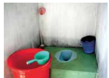
Typical pour-flush toilet connected to a septic tank
