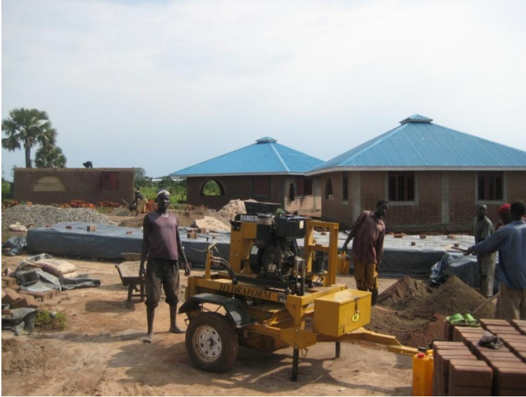
Block Moulding with Hydro form Machine on site.
