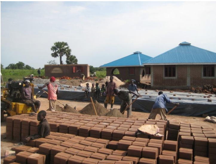
The ongoing construction of child development centre at Lira.
