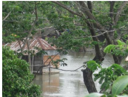
A village shop is under water
