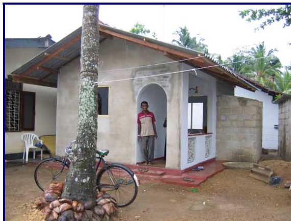
FIGURE 9: RECONSTRUCTION IS UNDERWAY IN SRI LANKAN COMMUNITIES
