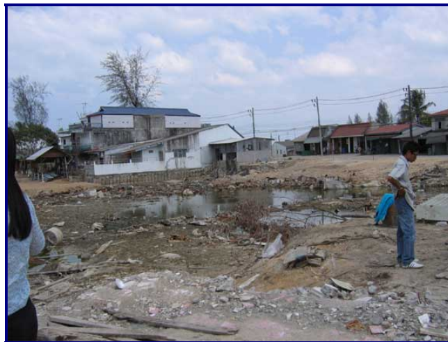
FIGURE 15: HOUSES, SCHOOLS, AND INFRASTRUCTURE COMPONENTS WERE DESTROYED BY THE TSUNAMI
