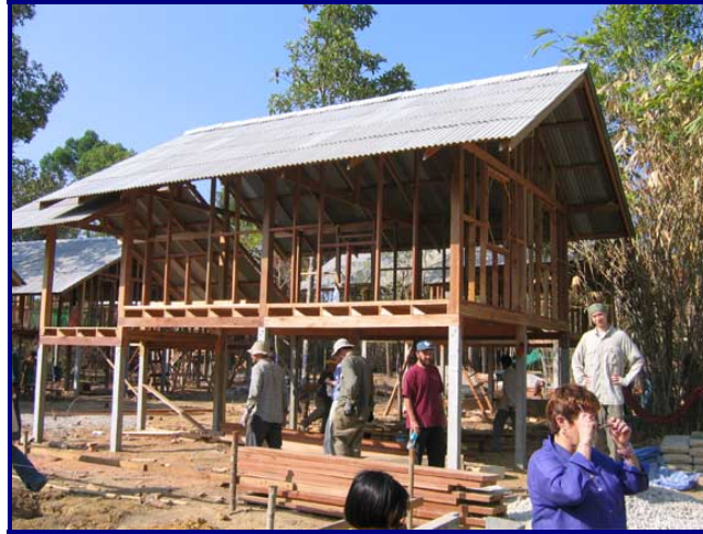
FIGURE 14: WORKERS HELP TO BUILD BACK BETTER
