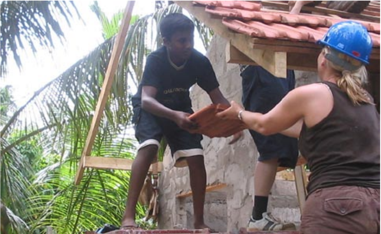
Rebuilding Together: Freshfields Buckhaus Deringer Employees work with local family members to build new houses for them in Hikkaduwa, Sri Lanka (Photograph courtesy Freshfield Brukhaus Deringer)
