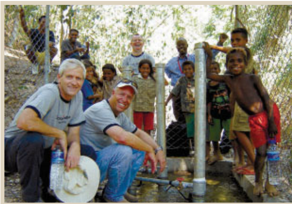
Construction of water pumps in rural Timor-Leste gives these communities easier access to clean water.
