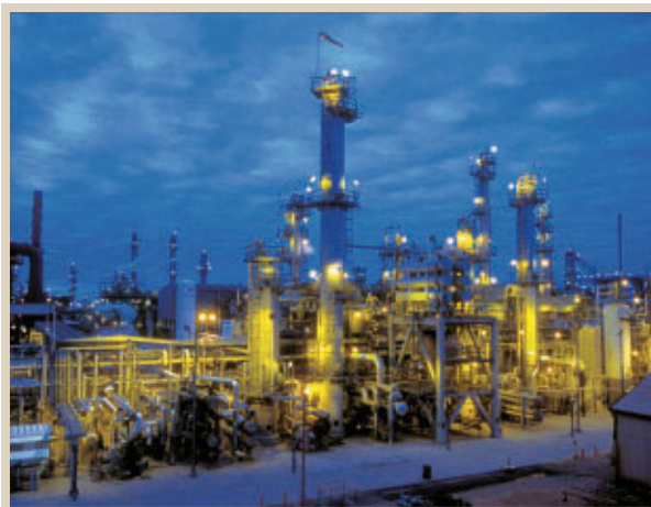
At the Borger refinery in Texas, our clean fuels investment was expanded to include installation of a new coking unit, due online in 2007. While enabling ULSD production, it also will allow the processing of heavier Canadian crude oil and a reduction in SO 2 emissions.
