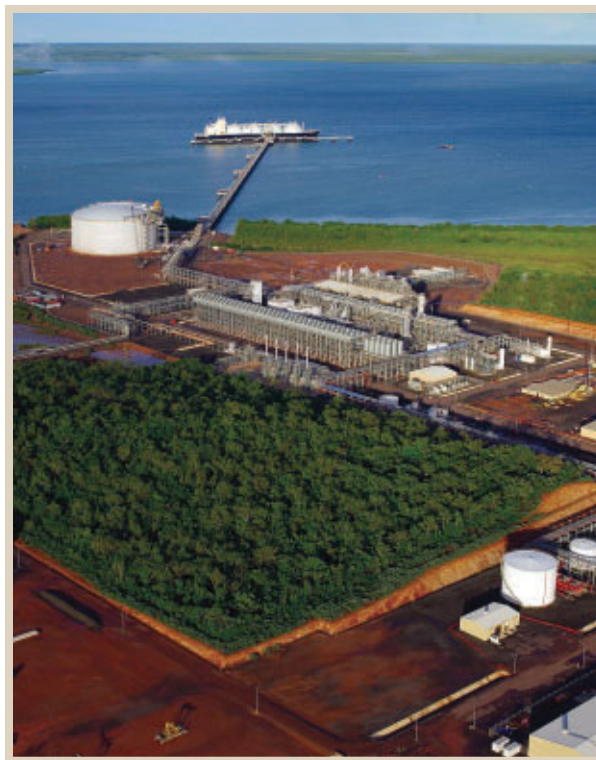
The Darwin LNG Facility.
