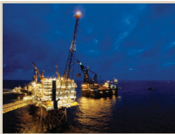
Installation of the CTour® purification process onto the Ekofisk platform.
