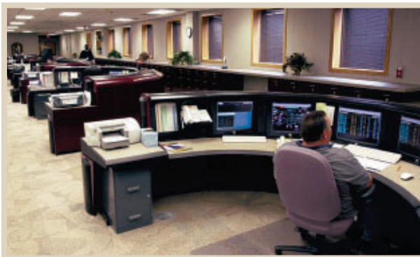
The control center in Ponca City, Oklahoma, uses a computerized system to monitor more than 12,000 miles of pipe from one central location.
