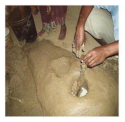
Third stage demonstration of firewood saving stoves where the laid bricks were covered with the mixed material until the pale at the middle was leveled. Then the pale was removed meaning that it was done.
