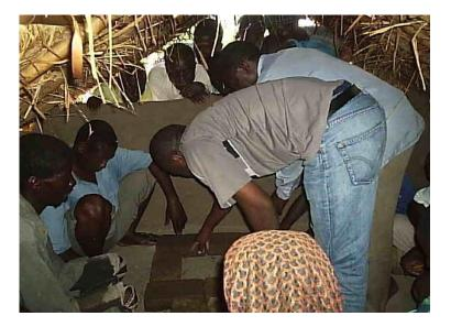
Second stage demonstration of firewood saving stoves where bricks were laid down in readiness for applying the mixed material.
